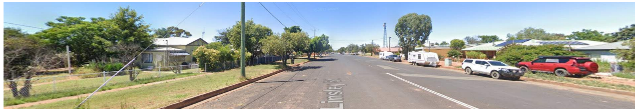
Figure 36: View 8 Linsley Street Looking South
