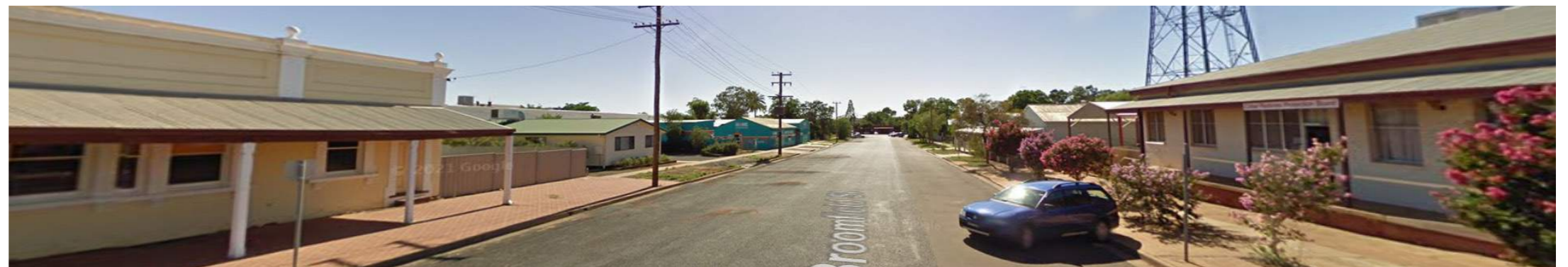
Figure 31: View 4 Broomfield Street Looking East
