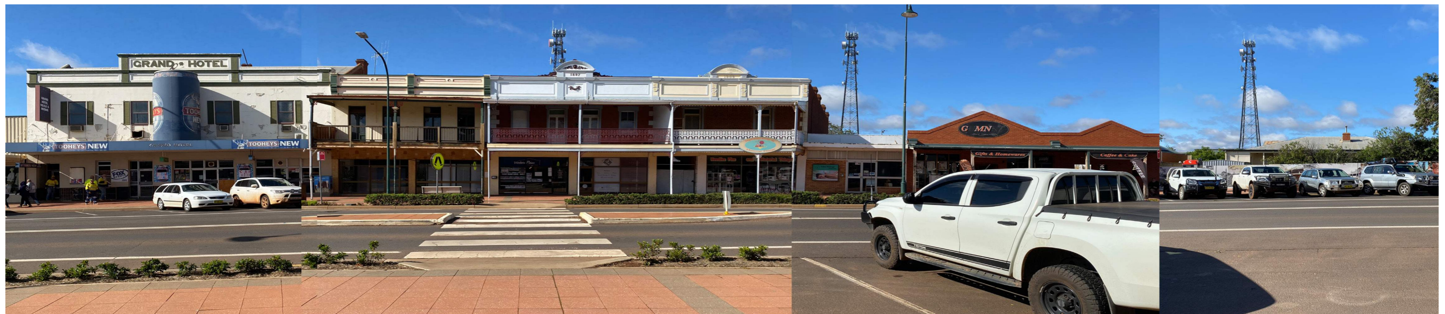
Figure 77: Existing Facade Elevation
