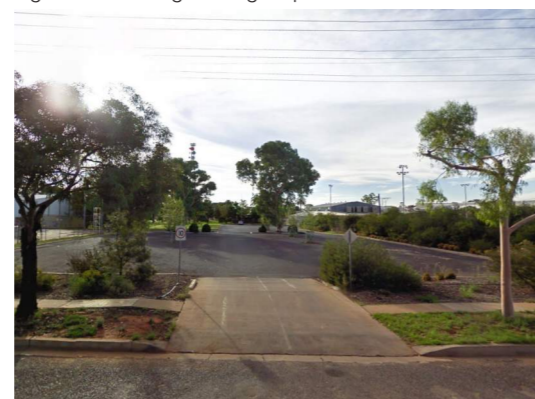
View 1: Parking Lot
