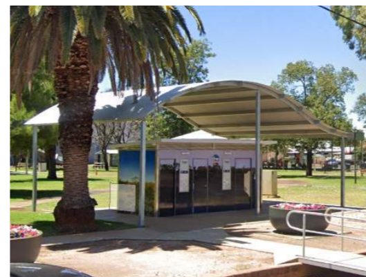
View 2: Drummond Park Public Toilets
