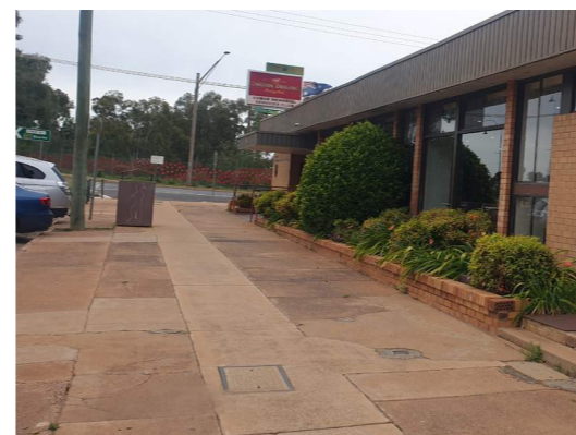
View 2: Older Concrete Footpath
