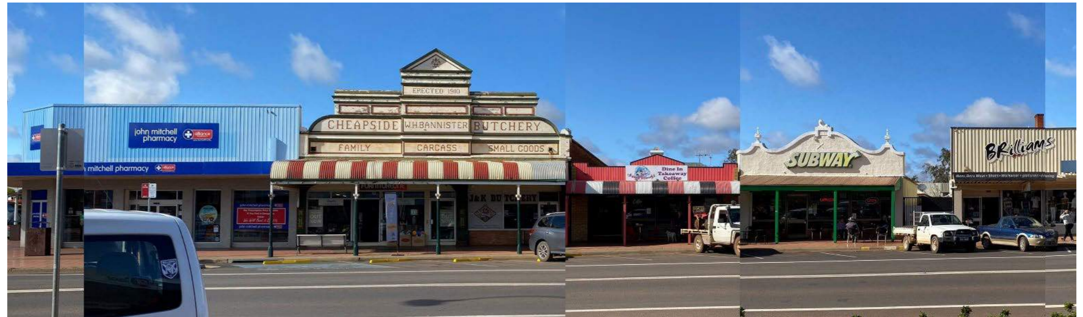
Figure 76: Existing Facade Elevation
