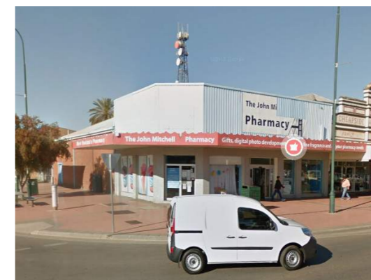
View 3: Pharmacy Building Awning
