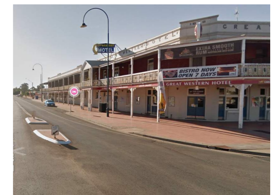
View 4: Motel Building Awning
