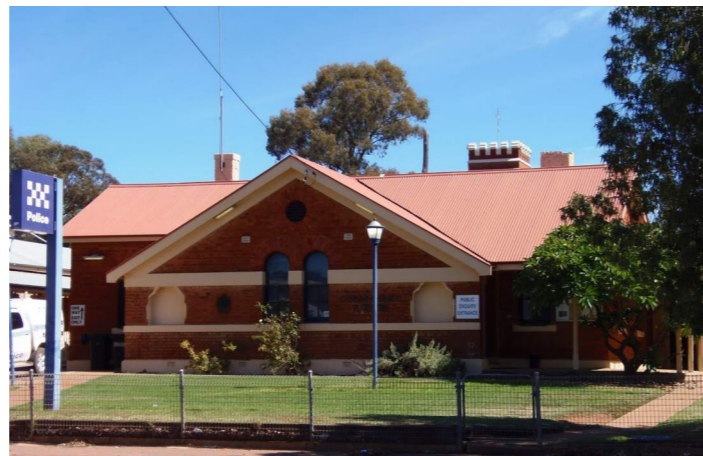
Figure 84: Cobar Police Station
